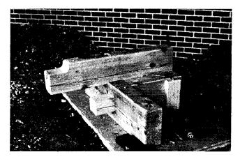
Fig. 3. Gamble House beams with additional pad attachment .
